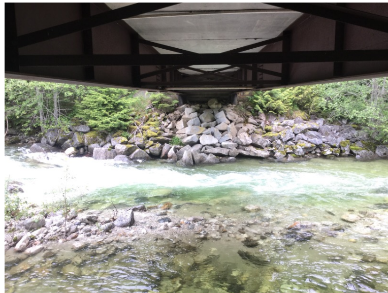
Left Bank Abutment when facing downstream
