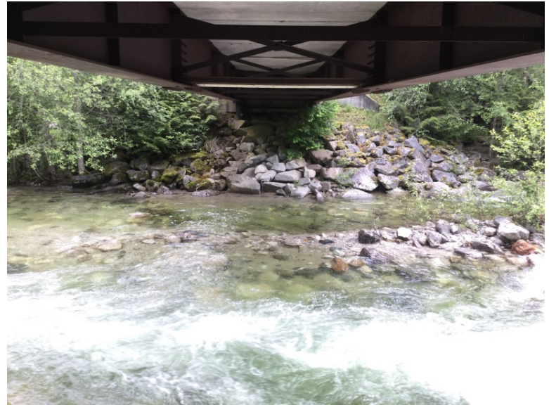
Right Bank Abutment when facing downstream
